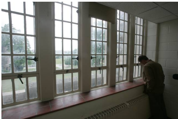
Figure 11. Typical Set of Windows in Norris Hall
